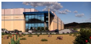
Diversified Data Center
