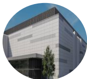
Diversified Data Center
